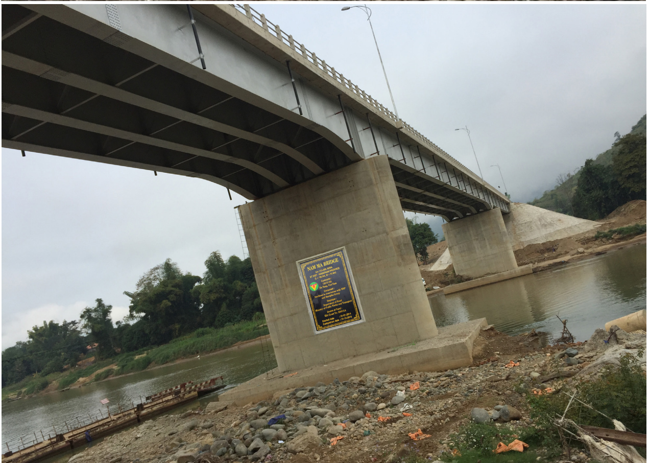
CONSTRUCTION OF 7 BRIDGES ON 6A NATIONAL ROAD HOUAPHAN PROVINCE – LAOS
