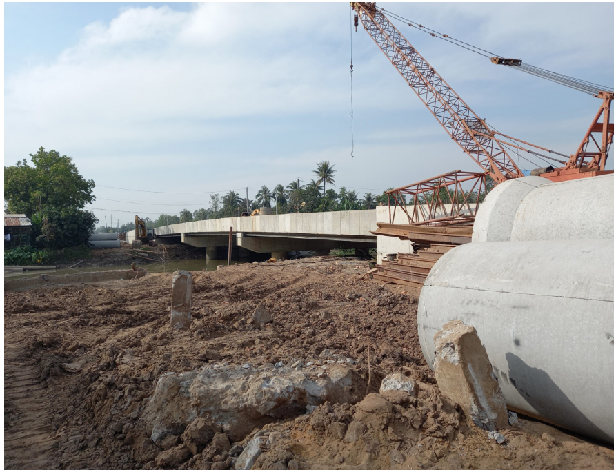
Transport Credit Project for National Road Network Improvement (Step 2, Phase 1) Balanced cantilevered pre-stressed concrete structure
