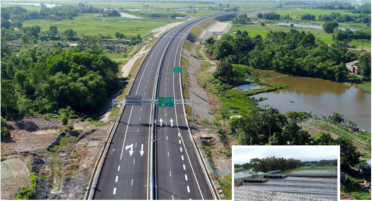
Package 01: Km0+00 – Km8+00 Bridge LRB02 Km02+460.75 across Yen River – Danang City Pre-stressed concrete structure L=33m
