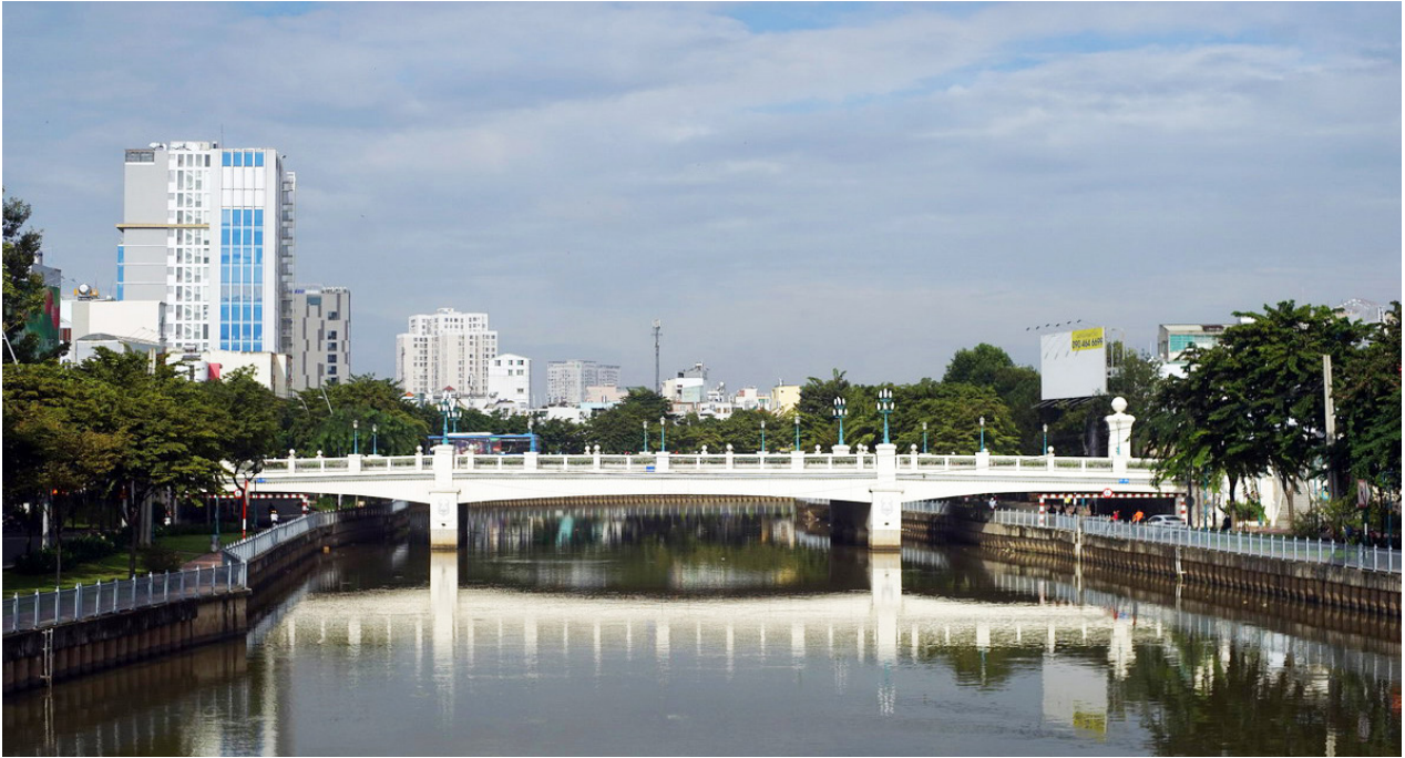
Project for Construction of 4 Bridges: Le Van Sy Bridge, Kieu Bridge, Bong Bridge on Nieu Loc - Thi Nghe canal Hau Giang Bridge on Tan Hoa - Lo Gom
