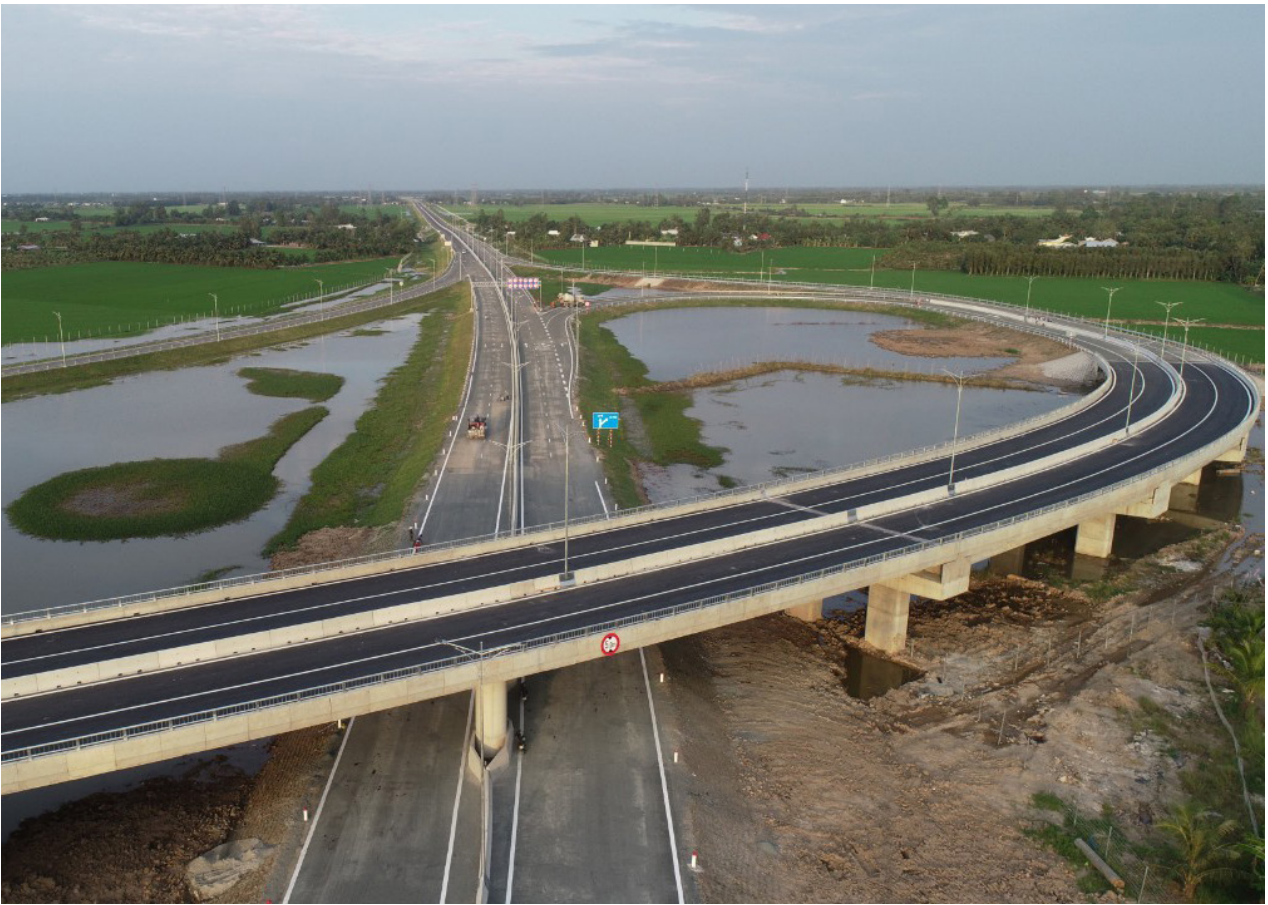
Construction Project of Lo Te – Rach Soi – Kien Giang Province
